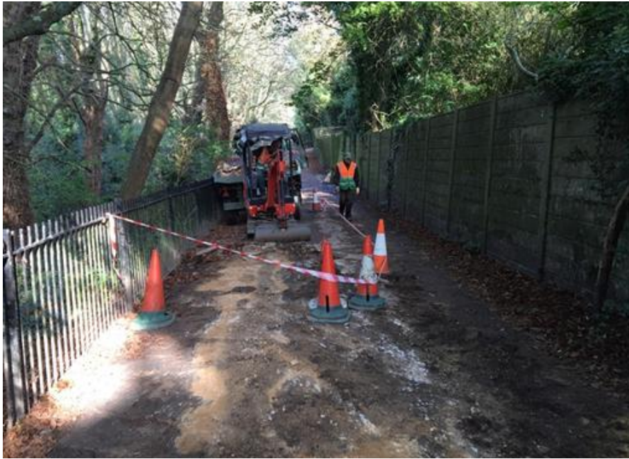
Figure 3: Conservation Team undertaking repairs to Millfield Lane
